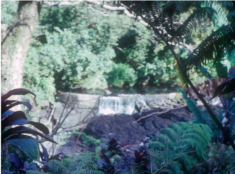
Concrete weir (mentioned in Overview) which “partially” diverts water from Palauhulu Stream for taro patches (lo‘i)..
