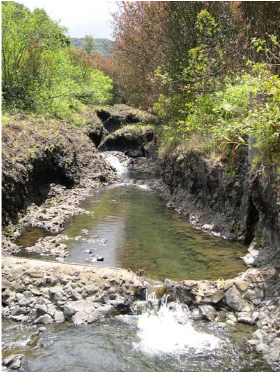
Left - View upstream from this site (SBN dk065r-040108). Note old concrete weir in lower portion of photo and just above remnants of concrete gauge on the right.
