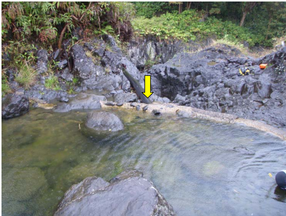
View downstream of diversion pool site gh063r-040208. Black 6" PVC pipe (yellow arrow) in the middle is carrying water downstream. Upper reach Pi'ina'au Stream, Maui, Hawai'i.
